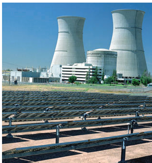
Solar array at shuttered Rancho Seco reactor—Clay Station, CA
