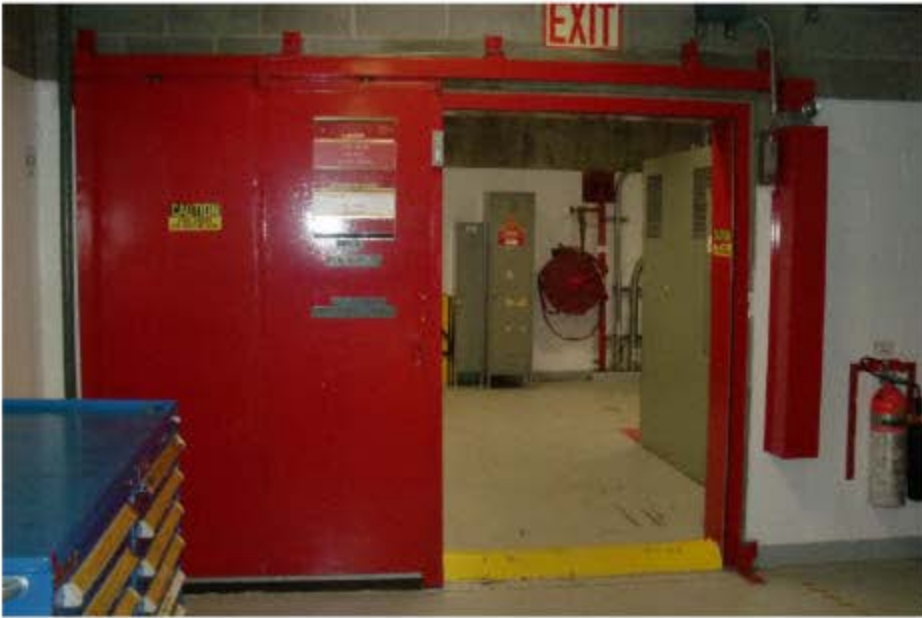
Pictured above is a fire door in its appropriate condition as per procedure and labeling.
