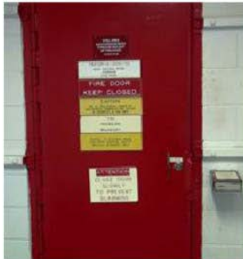
Pictured above is a vital area door that is designed to be kept closed following egress thru it. Note labeling – “Fire Door Keep Closed”
