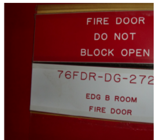
Fire Door Labeling - See page 2 f
